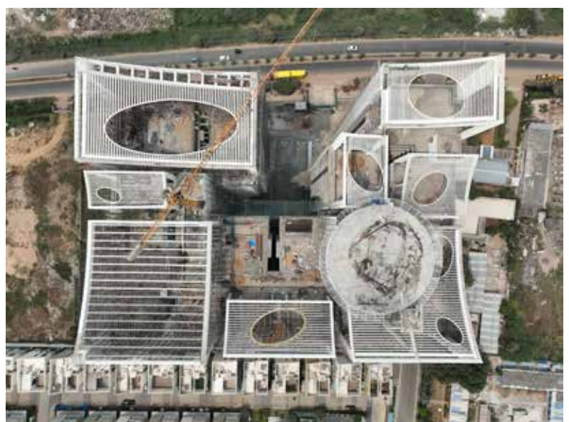
Current Site progress
